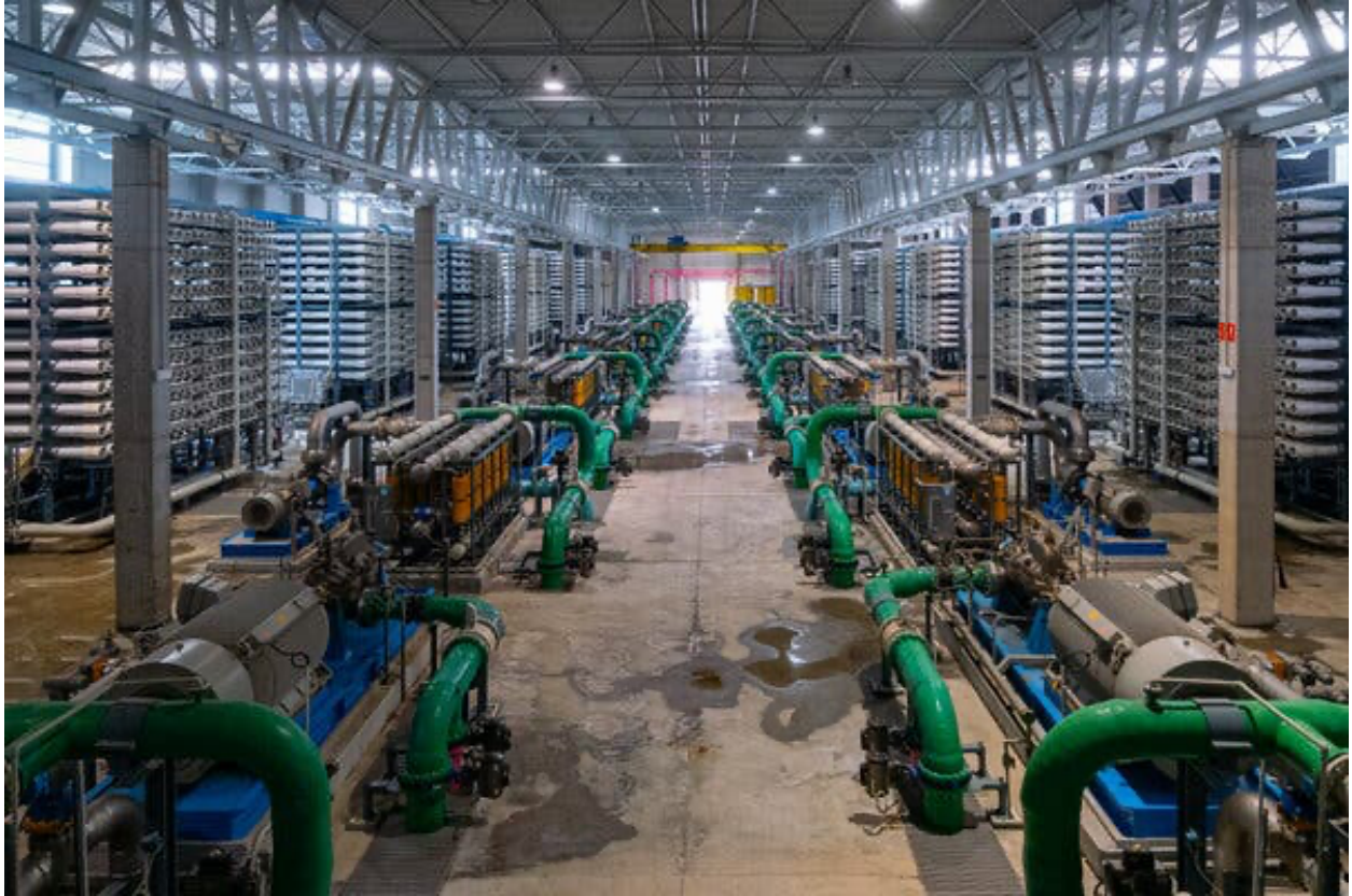
Part of the desalination plant where salt is removed from water through a process called reverse osmosis. Credit...Emilio Parra Doiztua for The New York Times
