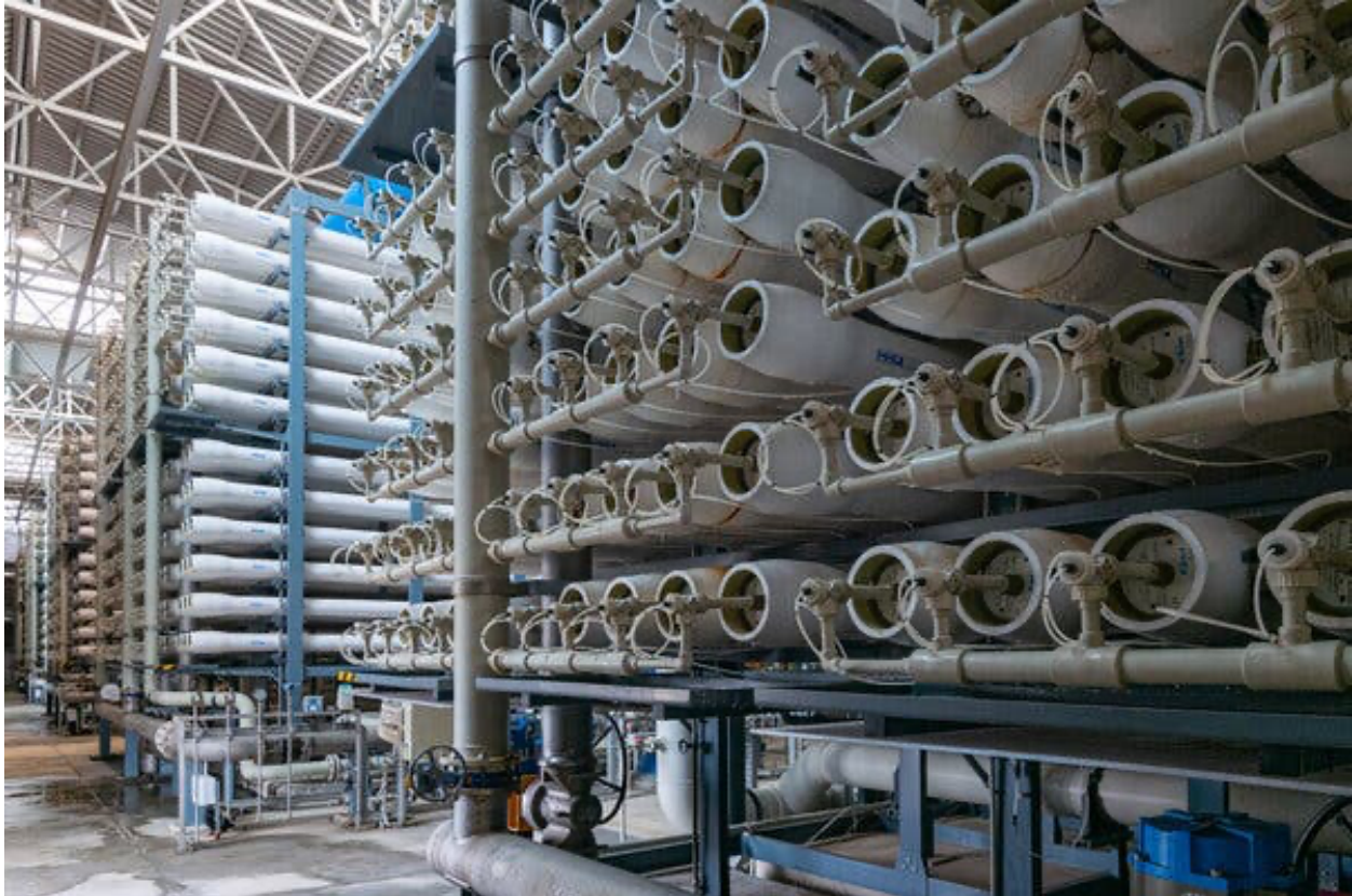
Stacks holding membranes used to remove salt. The costs of the technology are being lowered by using cheap solar energy.Credit...Emilio Parra Doiztua for The New York Times
